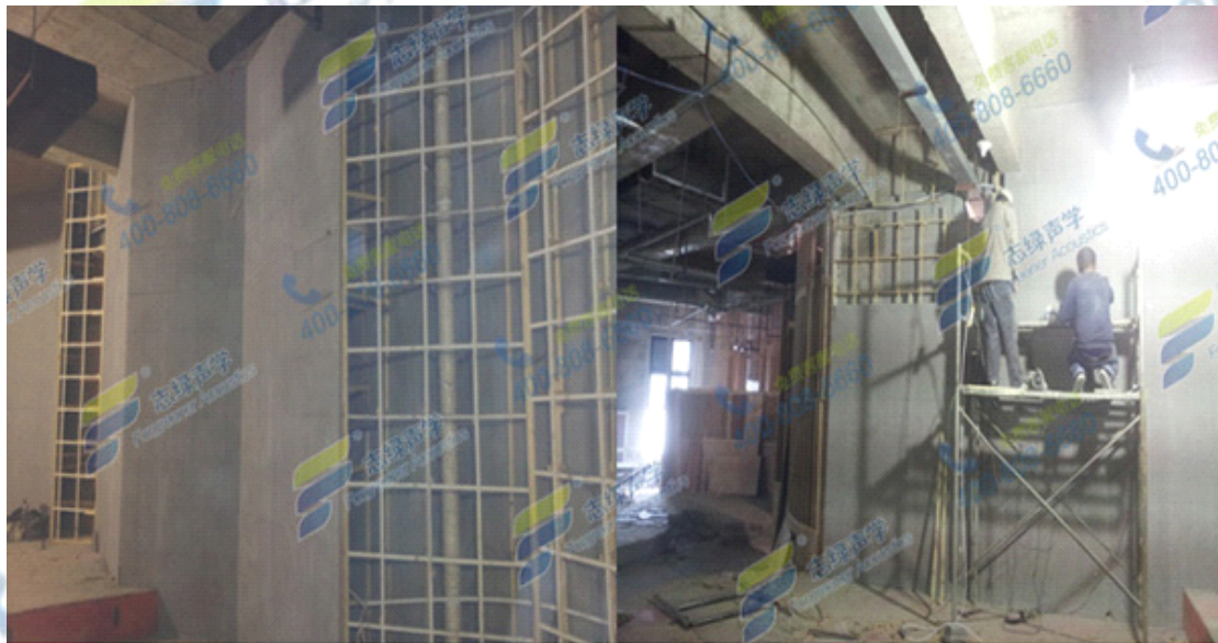
搭建木龙骨安装隔音板
